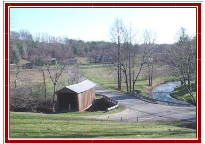
Jacks Creek Covered Bridge Route 615 Woolwine, VA
